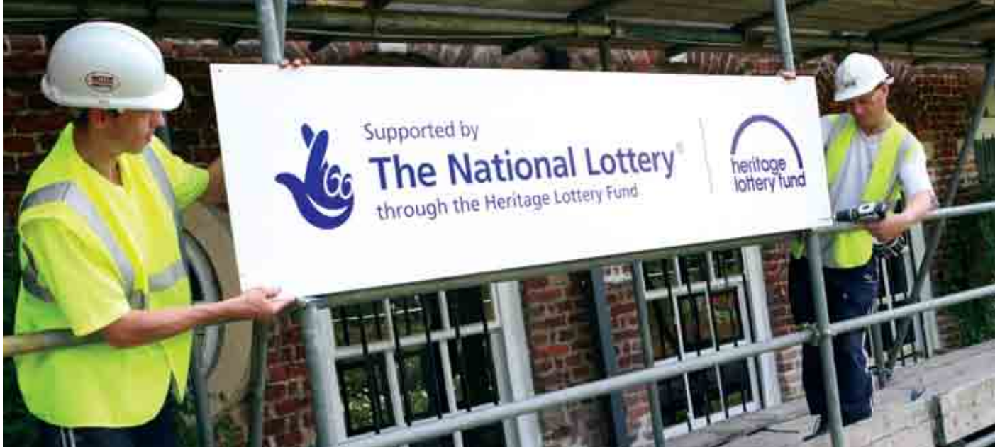
Installing a construction board at Hall Place, Bexley
