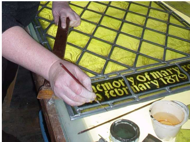
Stained glass restoration in progress
